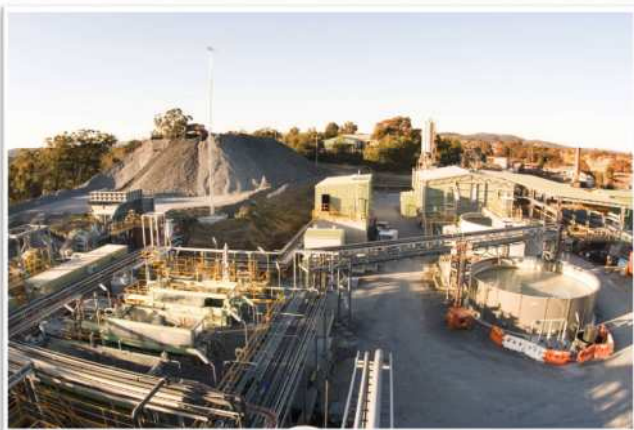
THE HILLGROVE ROM PAD VIEWED FROM THE CONCENTRATOR
