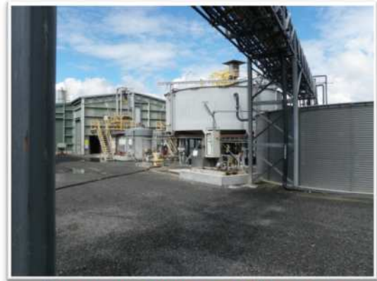
THE EXISTING THICKENER AT HILLGROVE
