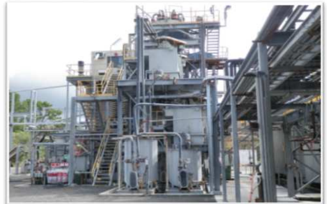
THE EXISTING CONCENTRATOR AT HILLGROVE
